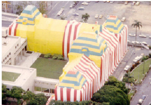
A large building enclosed in gas-proof sheets and fumigated to eradicate an infestation of drywood termites. The enclosure, which took three weeks to build, needed a total of 16 km of 2.5 m wide gas-proof sheeting.
