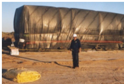
Sheeted fumigation of portable buildings.
