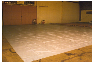
A gas-proof sheet is laid on a cracked (and leaky) godown floor to ensure that the enclosure will be gastight.
